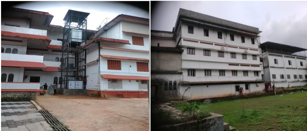
FIGURE 2: CAMPUS BUILDINGS VIEW
